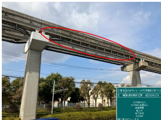
ひび割れ補修
