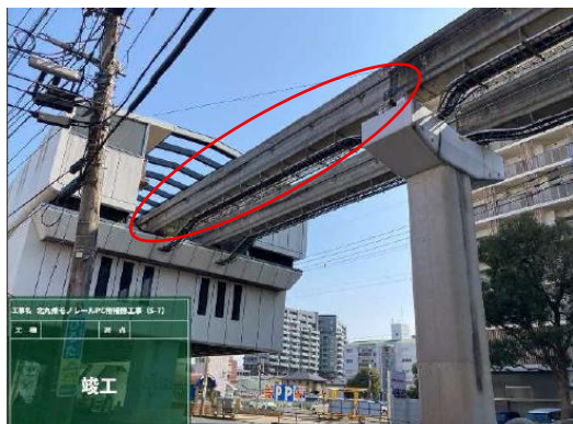
ひび割れ補修
